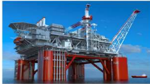
Energy (Oil & Gas, Wind Installation)
